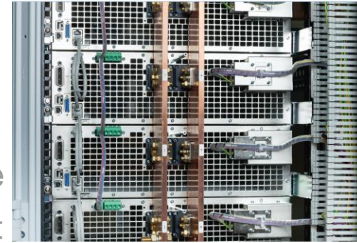
High current bus bar – system has lockable door
